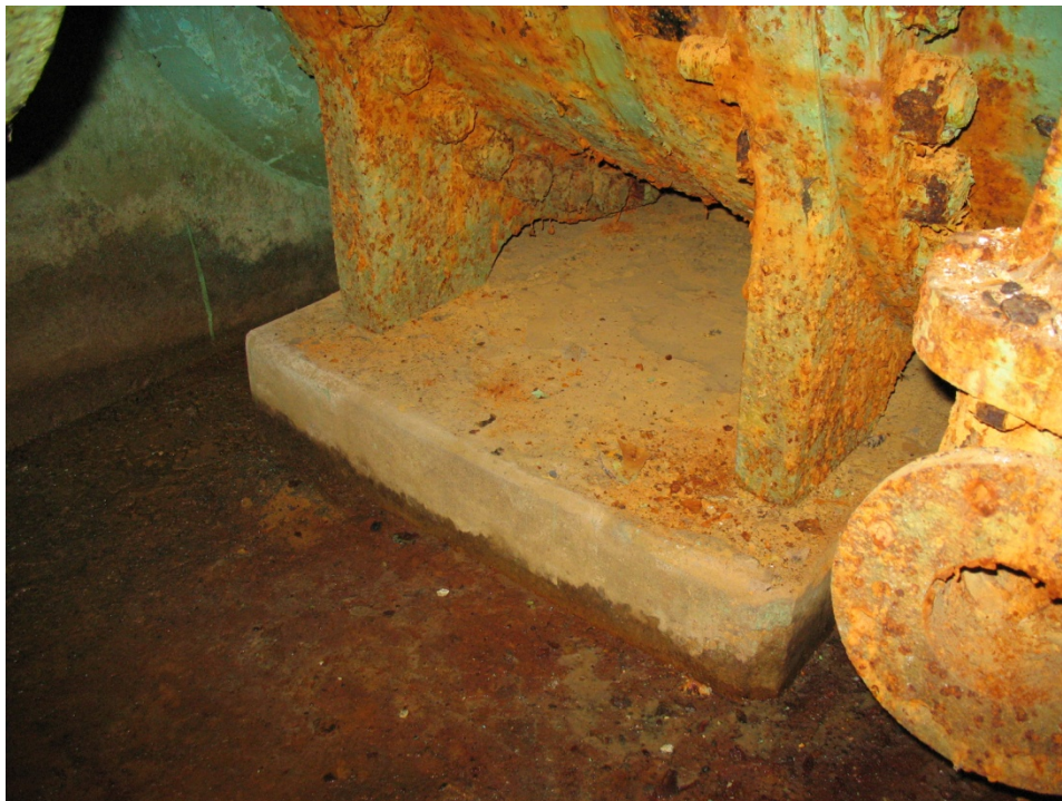
Figure 4 - Existing 1200 mm Valve Base Casting
