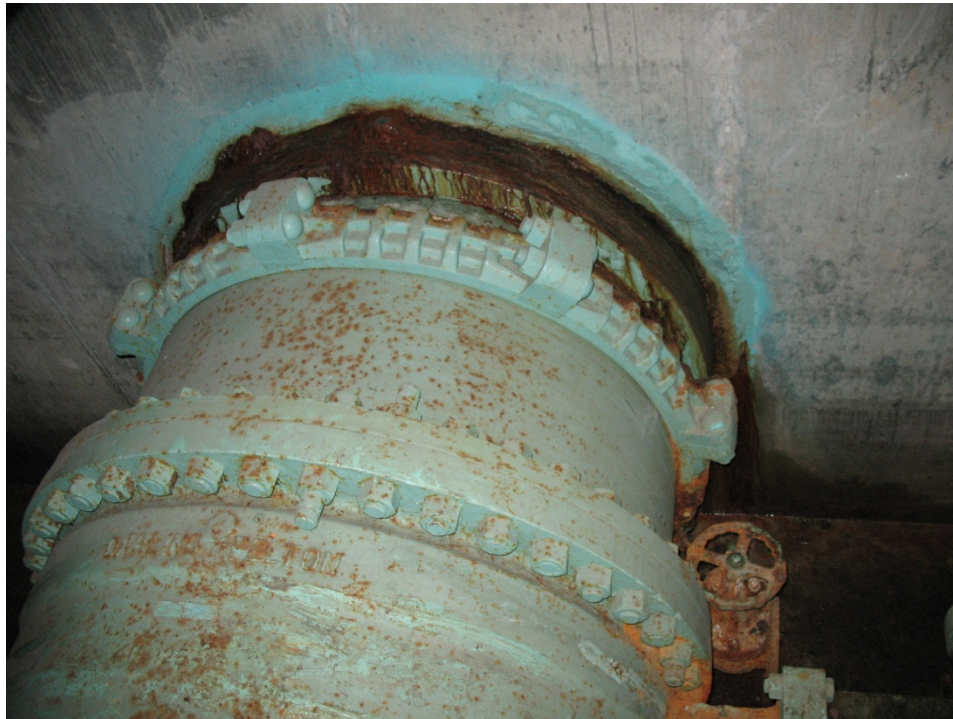
Figure 1 - Existing 1200 mm Spool and Style 44 Victaulic Coupling
