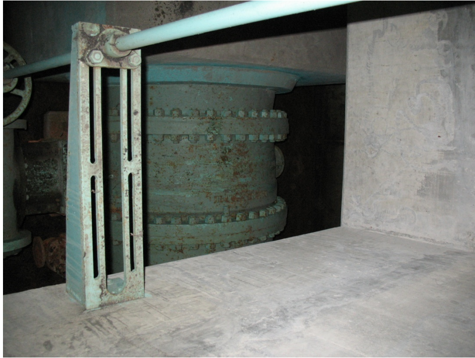
Figure 3 - Existing 1200 mm Valve and Stem Guide
